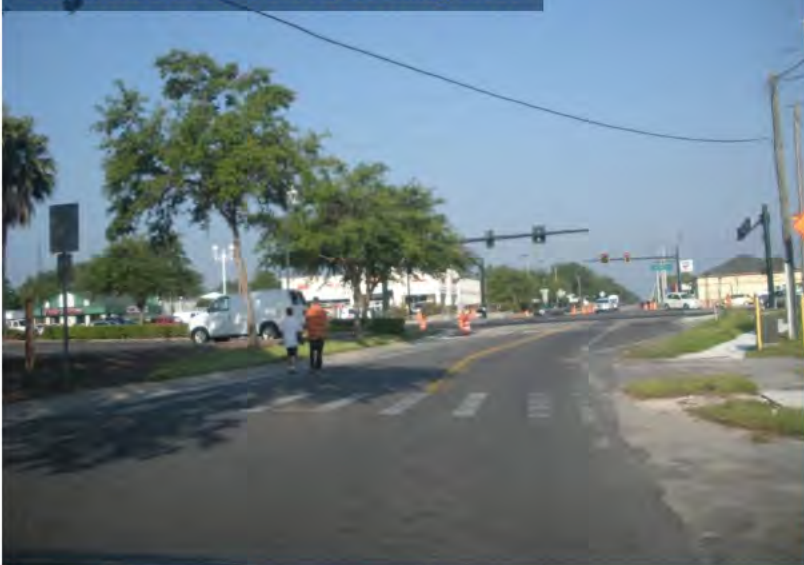
Griffin Rd East of US 441, Looking West
