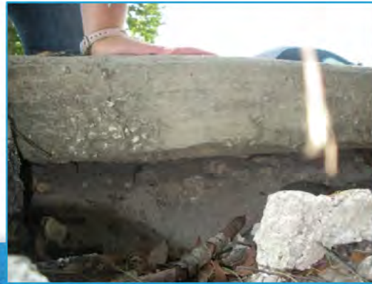
Drainage Issues at Southeast Corner
