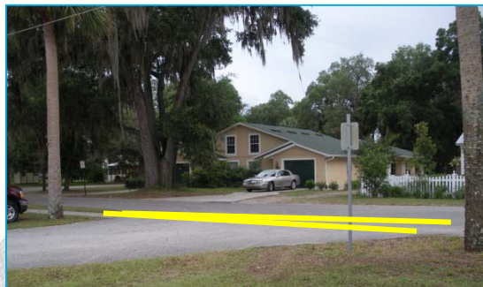
Missing Crosswalk at K-2 Carloop Exit
