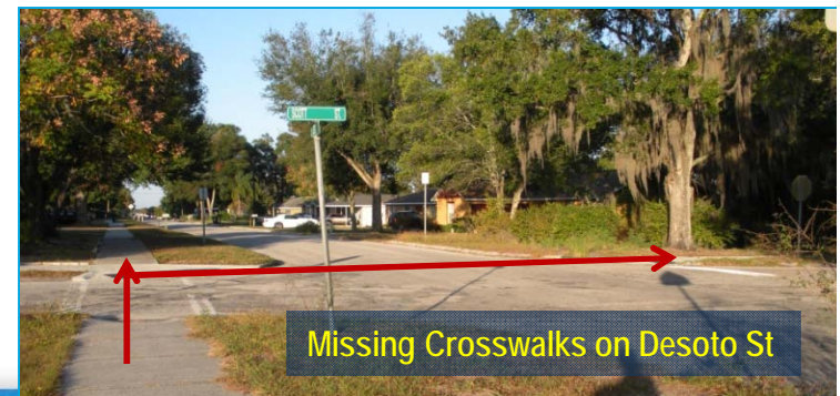
Missing Crosswalks on Desoto St
