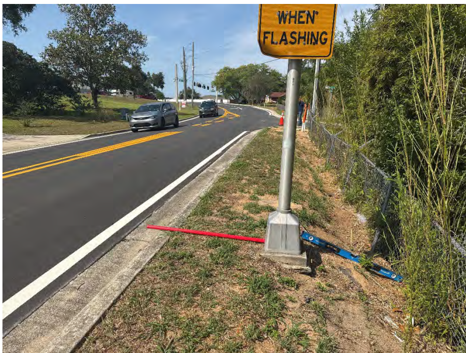
Photo ID: 67 / Date & Time: 5/9/2025 2:45:16 PM / Direction of View: Southwest
