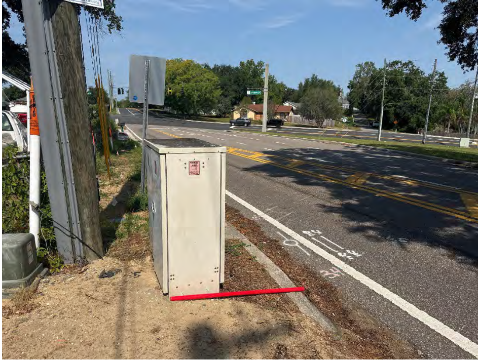
Photo ID: 69 / Date & Time: 5/9/2025 2:59:17 PM / Direction of View: West
