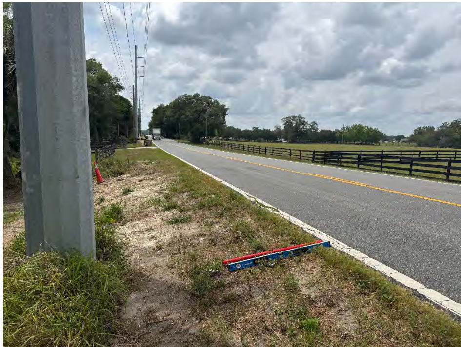
Photo ID: 44 / Date & Time: 5/8/2025 6:21:08 PM / Direction of View: West
