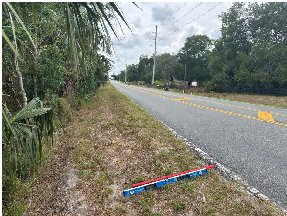
Photo ID: 42 / Date & Time: 5/8/2025 6:13:38 PM / Direction of View: West
