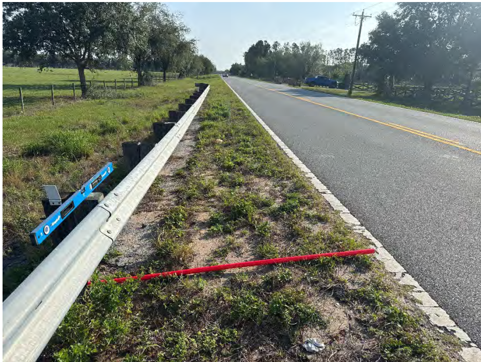
Photo ID: 46 / Date & Time: 5/9/2025 12:58:07 PM / Direction of View: Northeast
