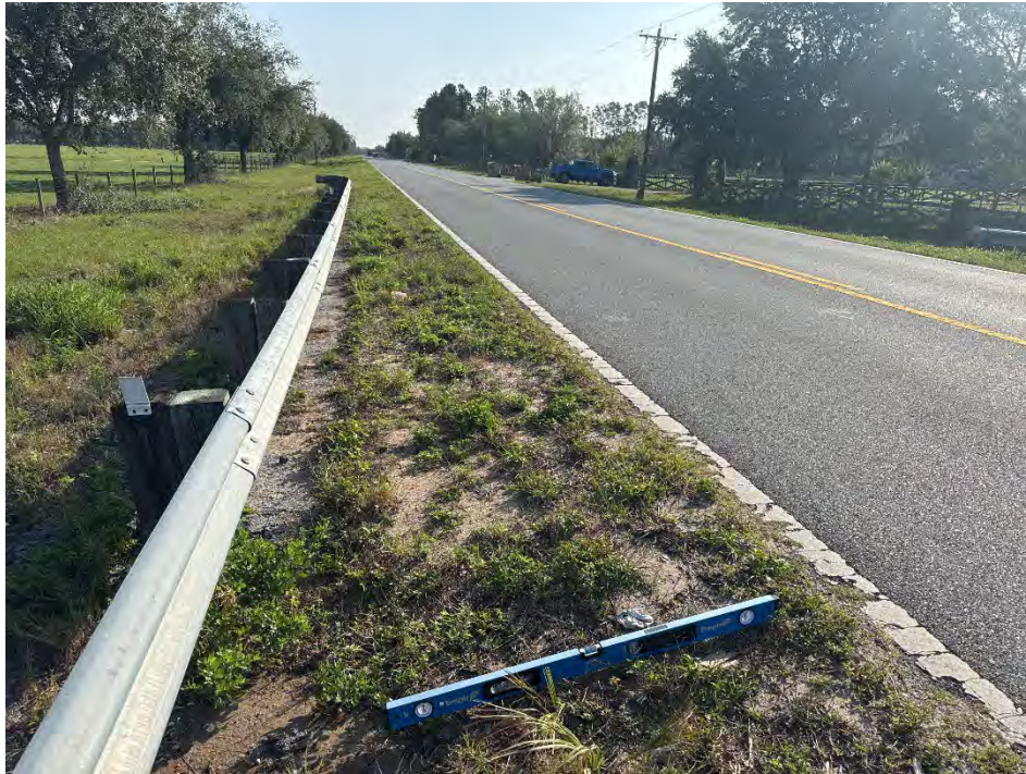
Photo ID: 45 / Date & Time: 5/9/2025 12:56:52 PM / Direction of View: Northeast
