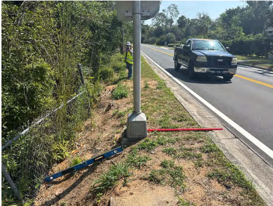
Photo ID: 66 / Date & Time: 5/9/2025 2:44:23 PM / Direction of View: Northeast
