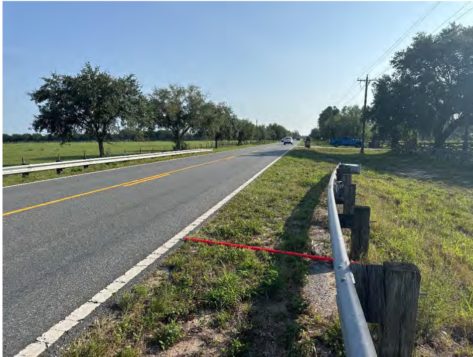
Photo ID: 47 / Date & Time: 5/9/2025 1:00:28 PM / Direction of View: Northeast
