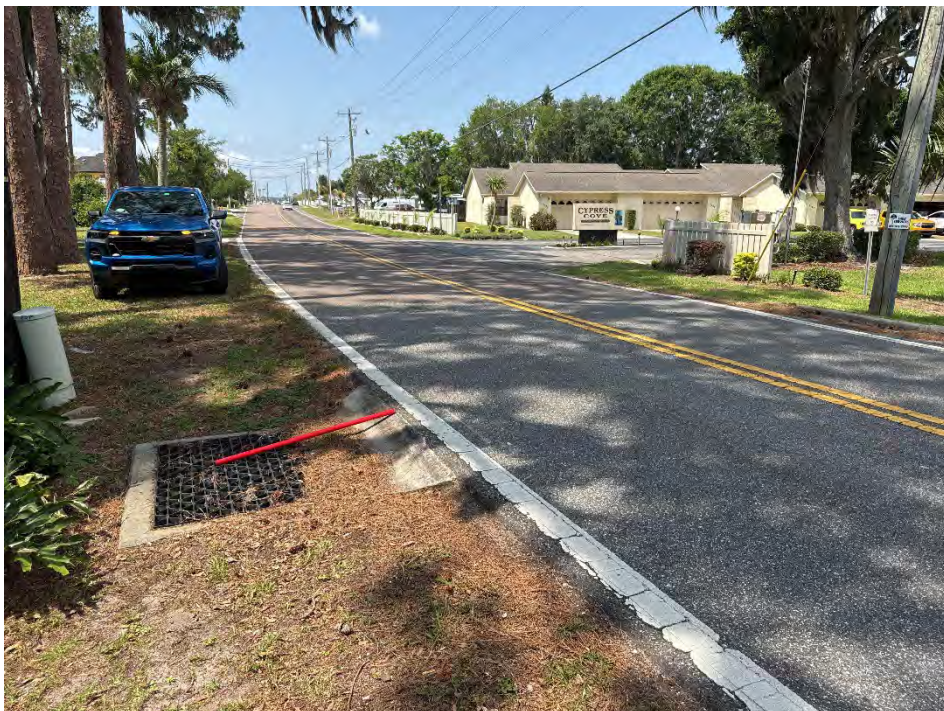
Photo ID: 26 / Date & Time: 5/8/2025 3:47:12 PM / Direction of View: Southwest
