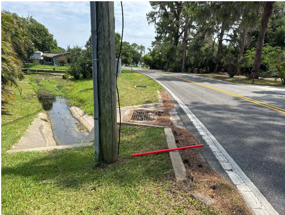
Photo ID: 27 / Date & Time: 5/8/2025 3:49:12 PM / Direction of View: Northeast
