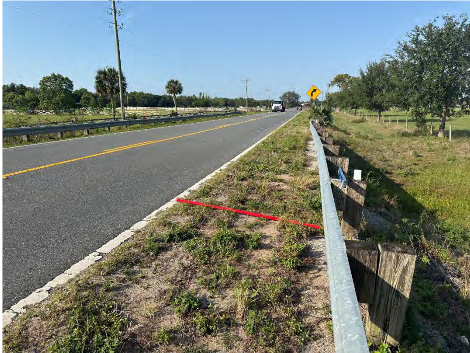
Photo ID: 49 / Date & Time: 5/9/2025 12:59:04 PM / Direction of View: Southwest
