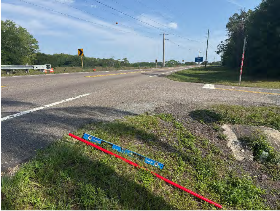
Photo ID: 59 / Date & Time: 5/9/2025 2:05:03 PM / Direction of View: Northwest
