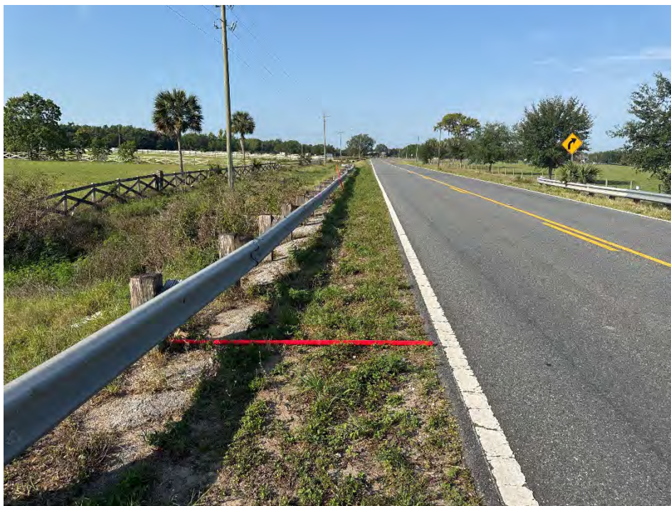
Photo ID: 48 / Date & Time: 5/9/2025 12:59:58 PM / Direction of View: Southwest
