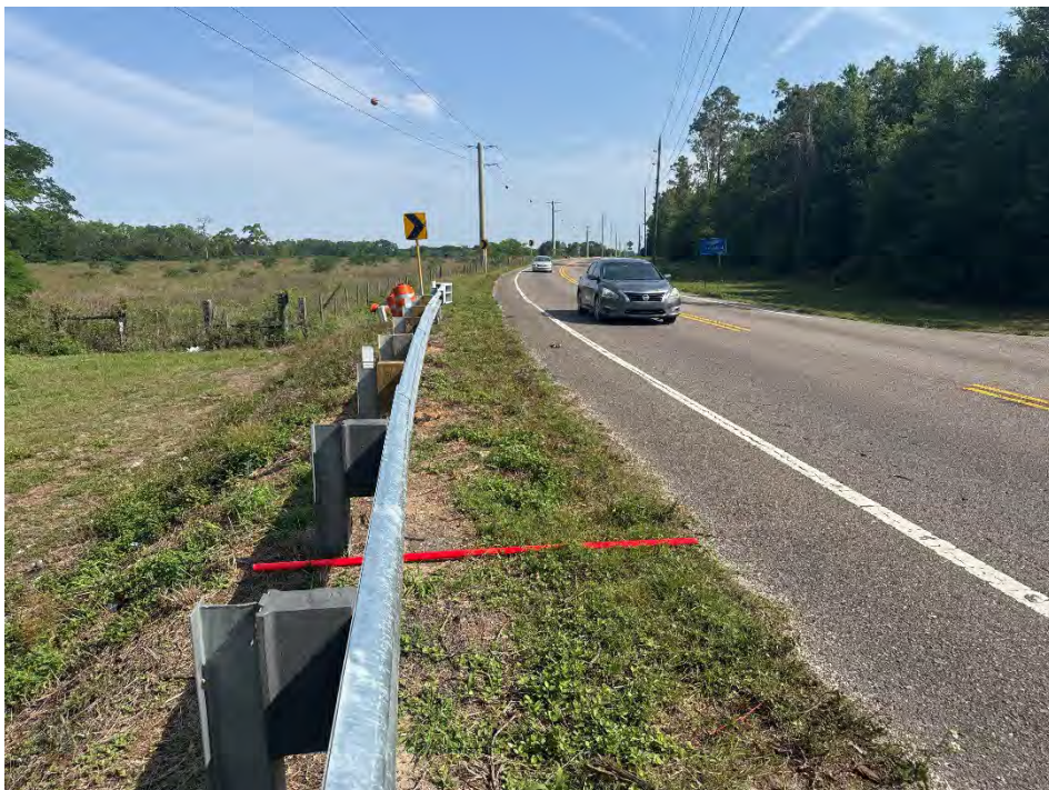
Photo ID: 60 / Date & Time: 5/9/2025 2:05:56 PM / Direction of View: Northwest
