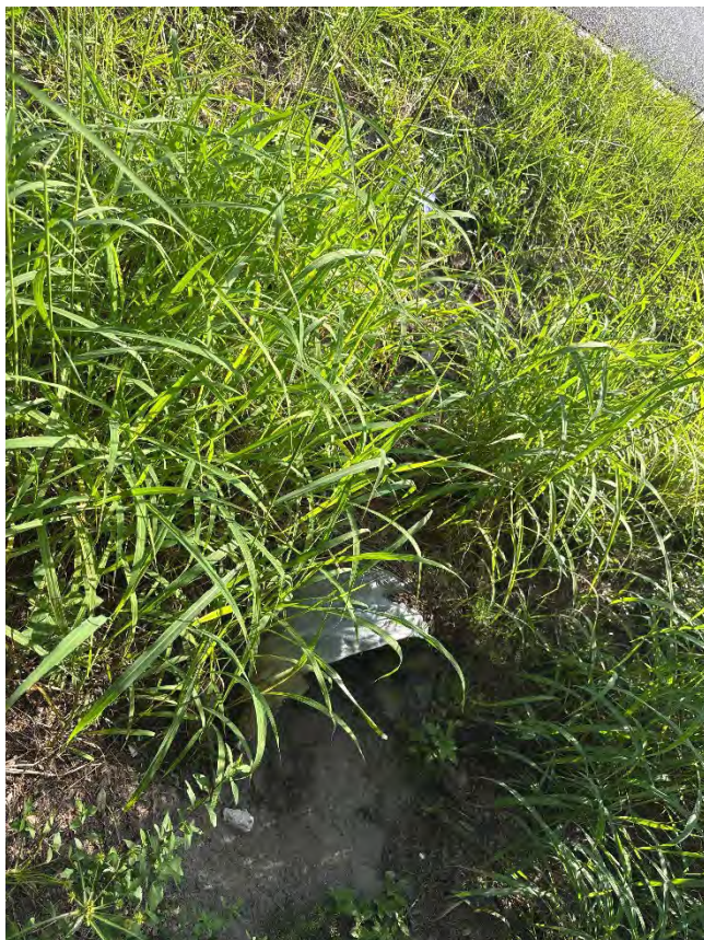
Photo ID: 81 / Date & Time: 6/10/2025 12:36:25 PM / Direction of View: North (Down)
