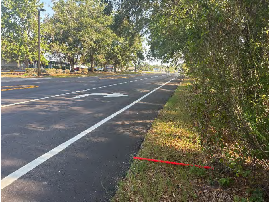
Photo ID: 50 / Date & Time: 5/9/2025 1:29:52 PM / Direction of View: North Northwest
