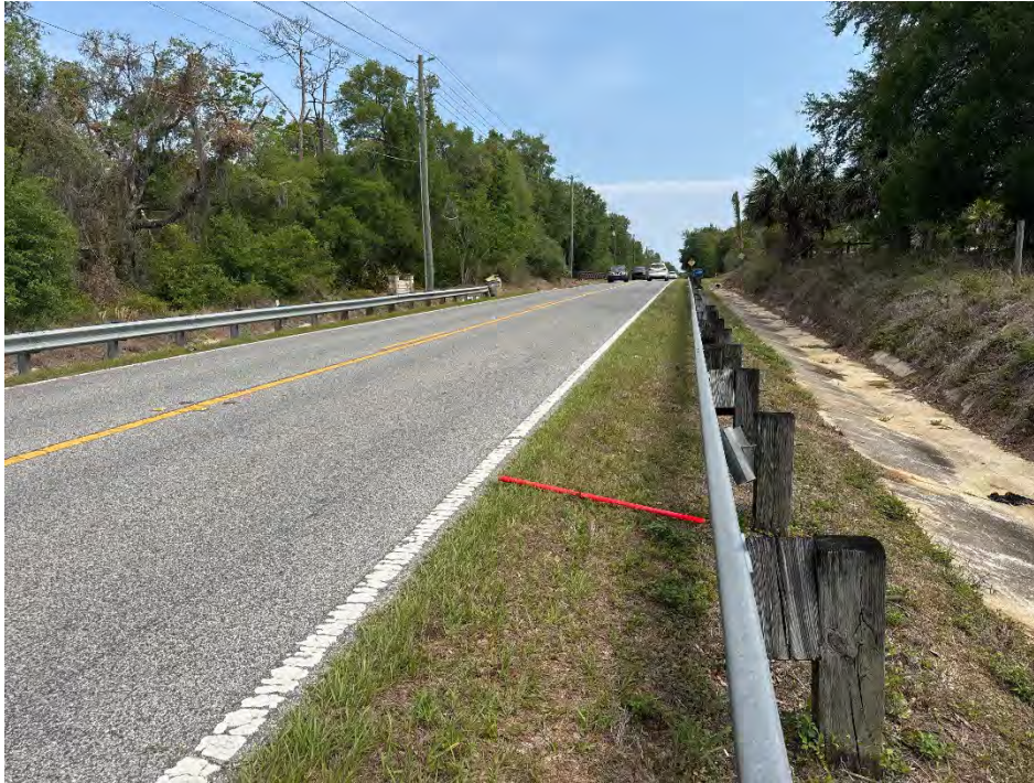
Photo ID: 20 / Date & Time: 5/8/2025 2:54:50 PM / Direction of View: North
