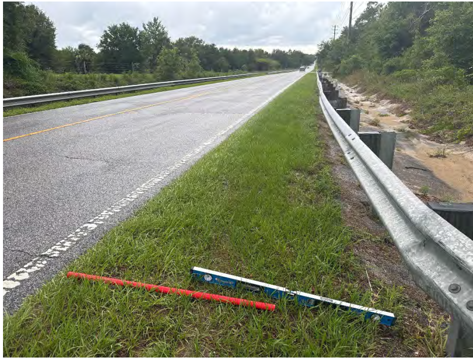
Photo ID: 92 / Date & Time: 6/10/2025 3:04:21 PM / Direction of View: North
