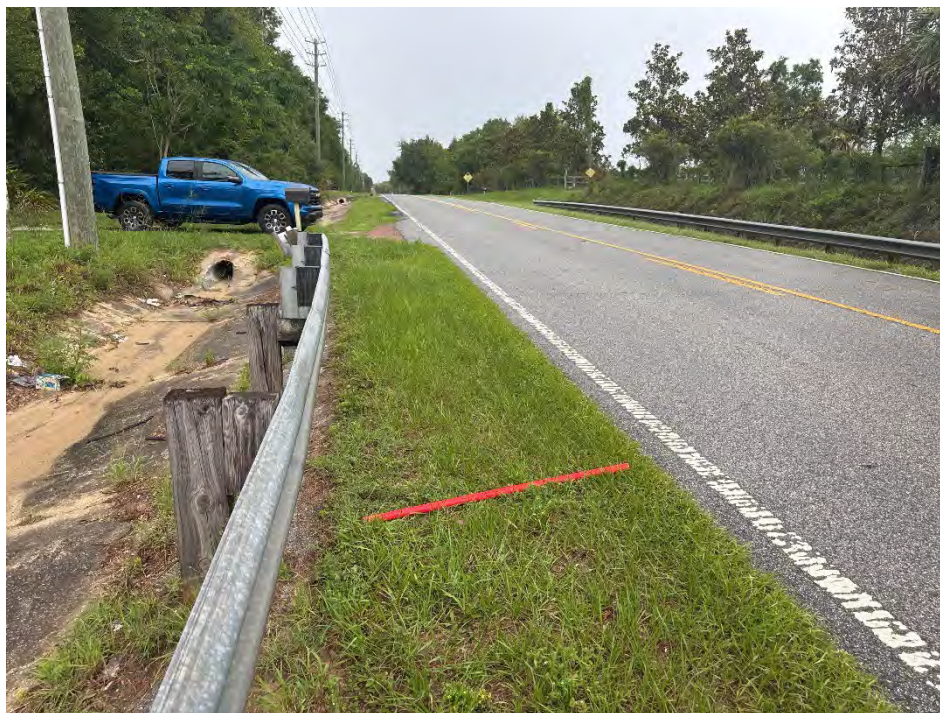
Photo ID: 93 / Date & Time: 6/10/2025 3:06:29 PM / Direction of View: South
