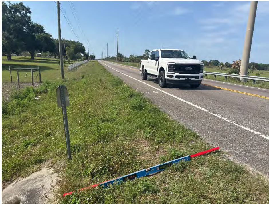
Photo ID: 64 / Date & Time: 5/9/2025 2:17:45 PM / Direction of View: South
