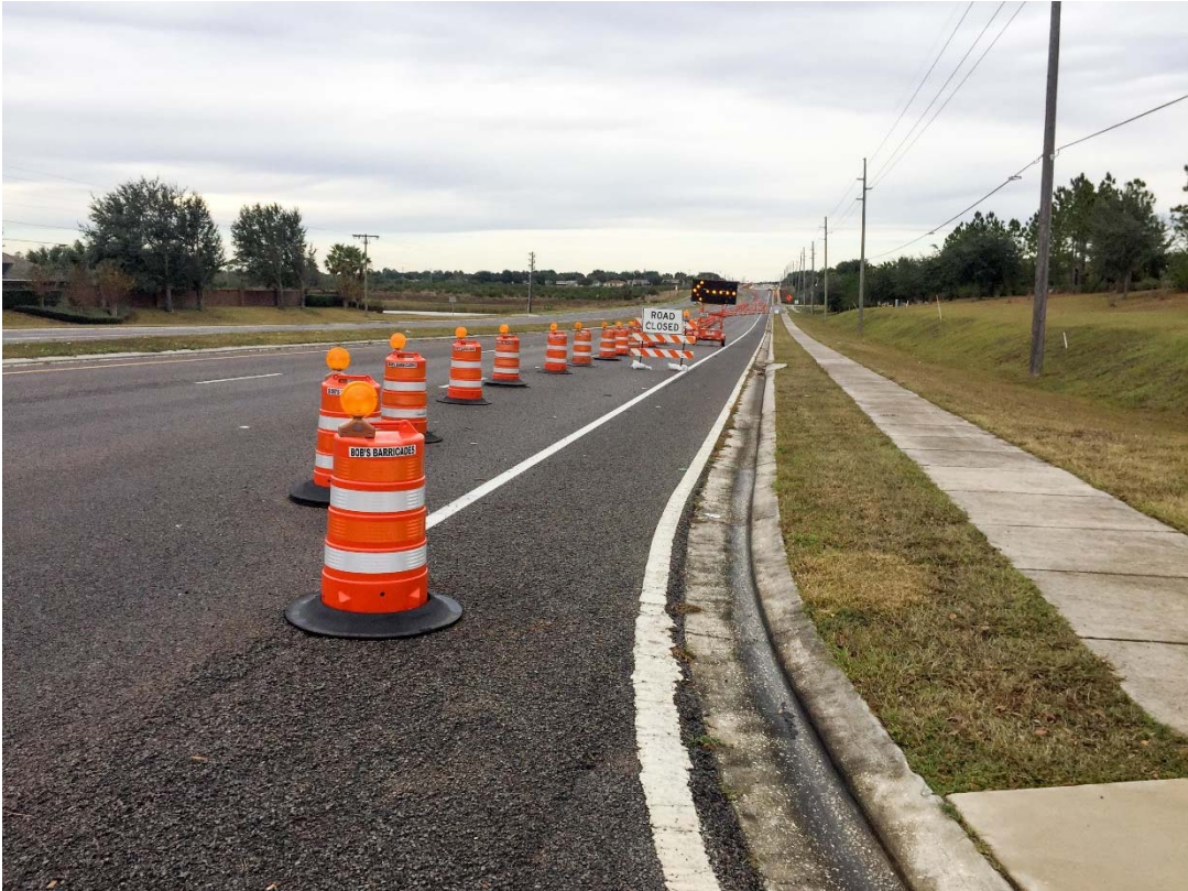
Photo 21: Holly Grove Blvd. looking Northwest at entrance of Orange Tree
